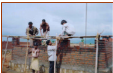
School under construction
