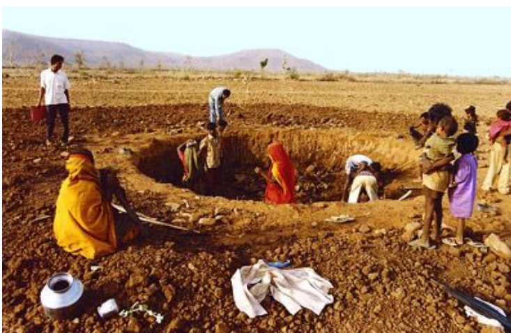
Irrigation well under construction at Village Agraa
